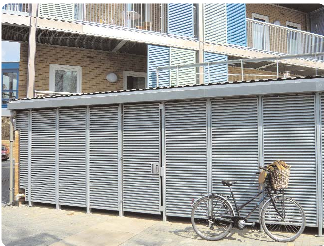
Figure 27: Secure cycle parking compound outside flats.
