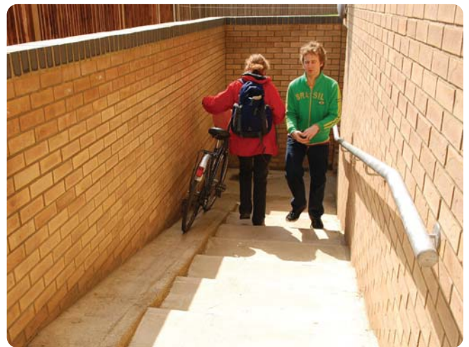
Figure 29: Steps and wheeling ramp giving access to communal cycle parking area. Two ramps would improve ease of use.
