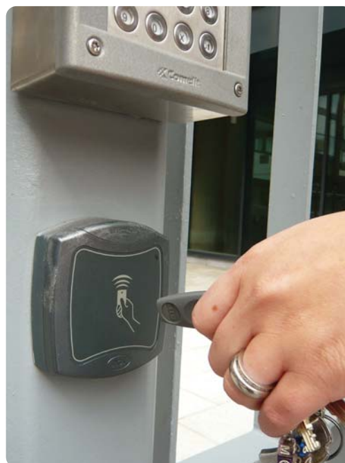
Figure 30 & 31: The use of smart card and proximity keys is recommended for secure access to communal sites, however, this needs to be well managed to remain effective.
