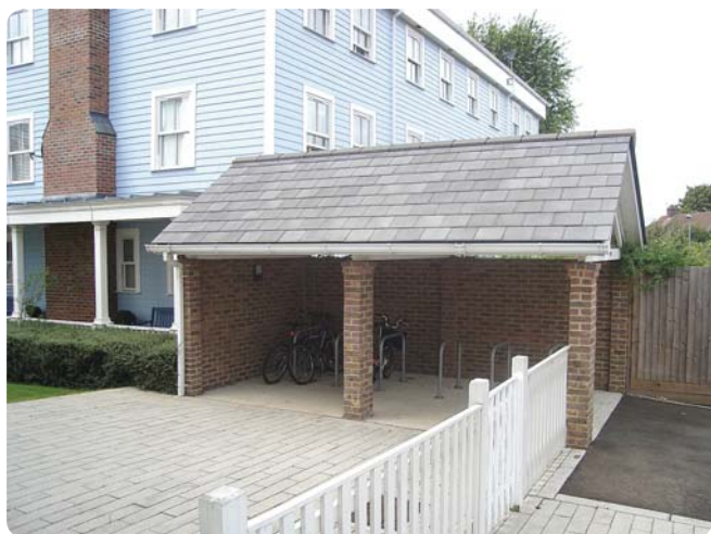
Figure 24: Good coverage provides protection from driving rain.
