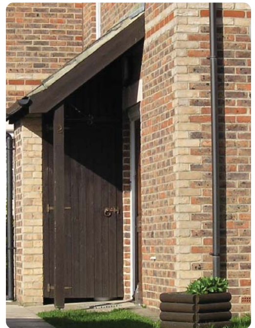
Figures 18 & 19: Cycle parking built into an extension of the porch: preferred approach (Note: doors should be wider and mortice locks fitted).
