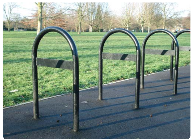
Figure 3: 'A' frame style stands are an acceptable variation and recommended where children's bikes may be parked.
