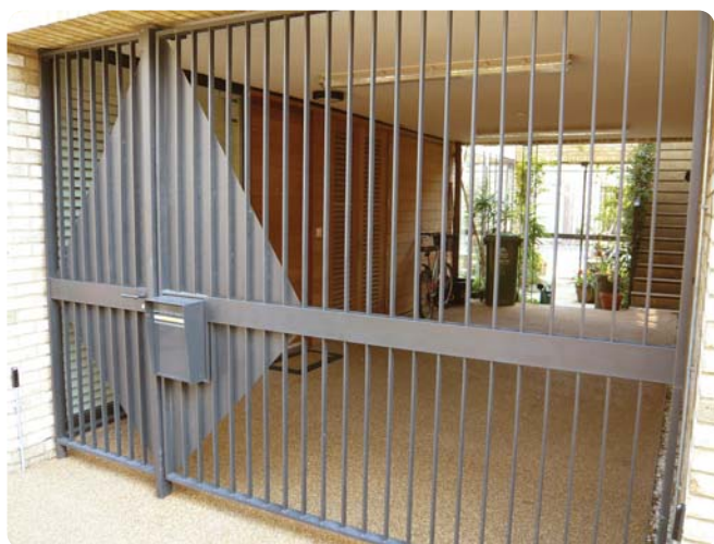
Figure 15: Secure parking for both cycles and car provided by the use of two gates.
