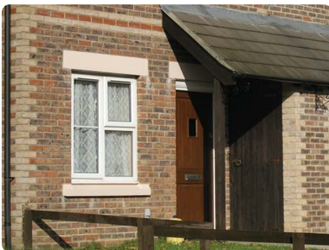
Figures 18 & 19: Cycle parking built into an extension of the porch: preferred approach (Note: doors should be wider and mortice locks fitted).
